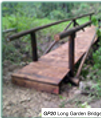
GP20 Long Garden Bridge
